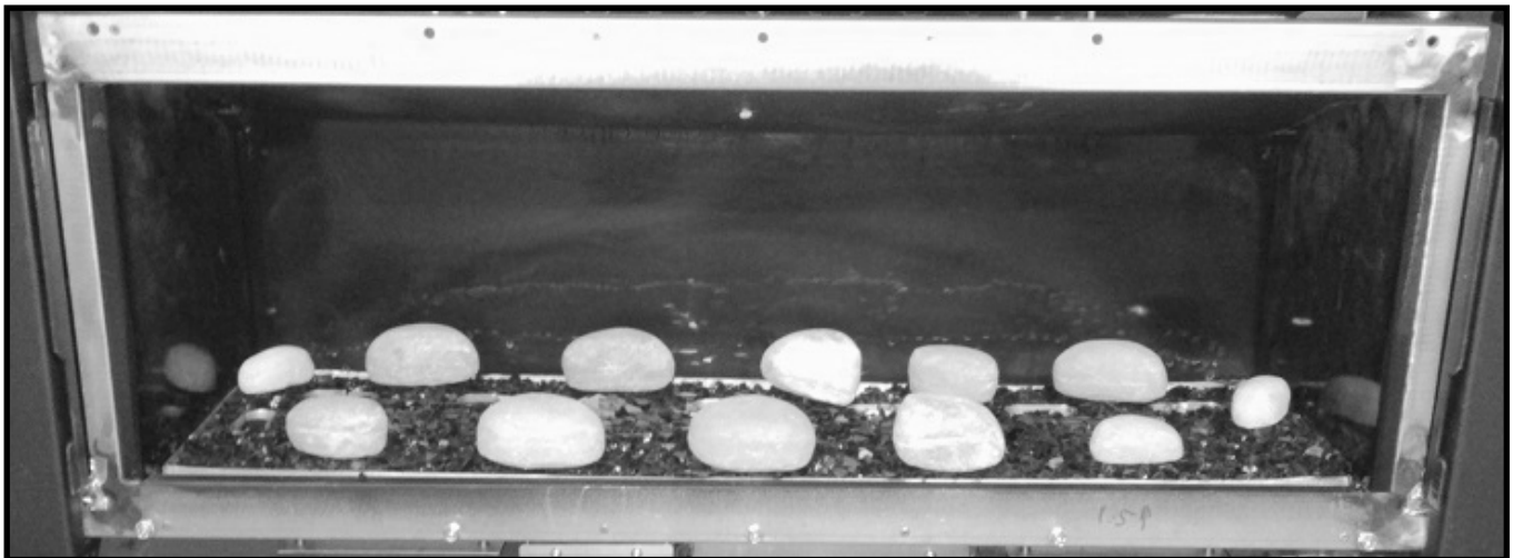
Figure 57: Rock set installation.
